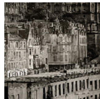
ST CHRISTOPHER INN DIVERSE ROOFSCAPE
