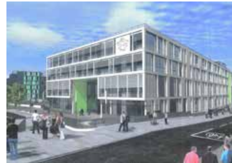
3 BOROUGHMUIR HIGH SCHOOL ON SITE
